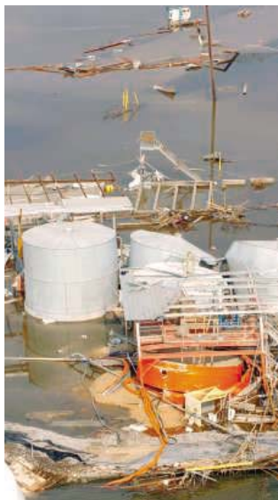
Damage to oil storage tanks in Cameron, Louisiana, caused by Hurricane Rita.
